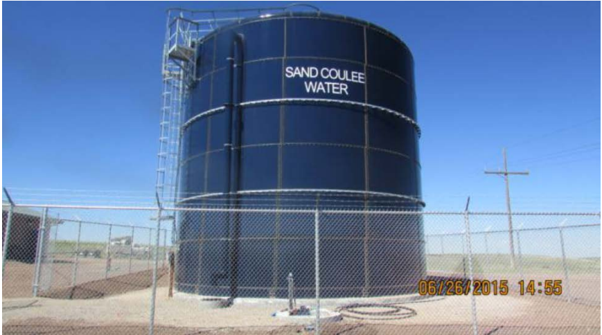
New water storage tank in June 2015
