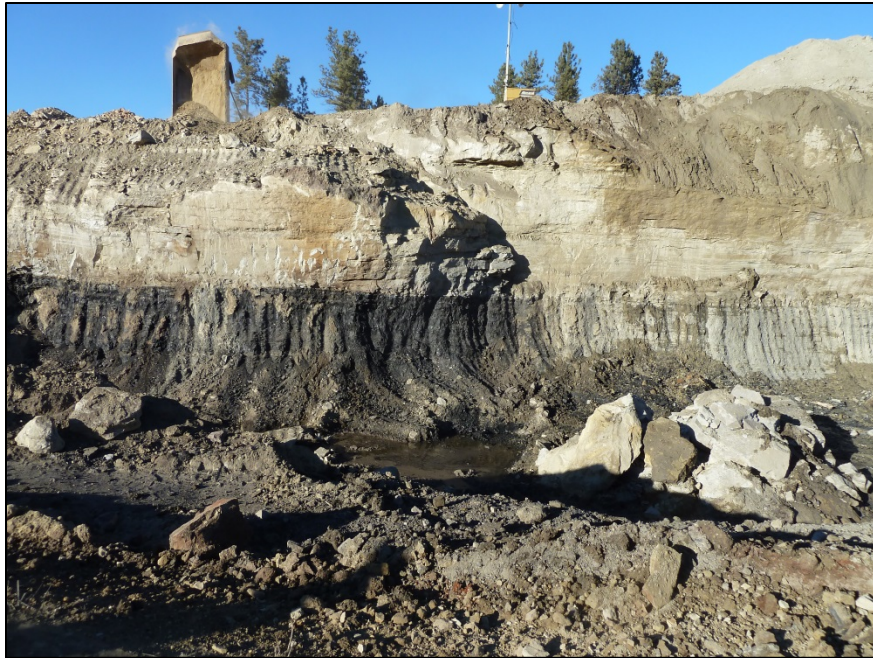
Excavation of burning coal seam (OSMRE site-visit, January 29, 2015)
