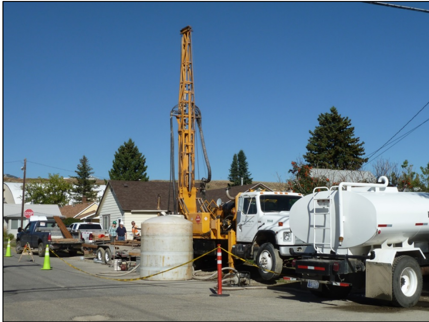
Drilling core samples (OSMRE site-visit, August 27, 2014)
