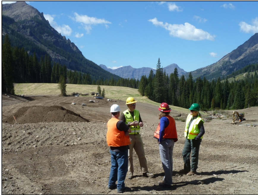
MT AML staff discussing the progress/status of the project (OSMRE site-visit, August 28, 2014)
