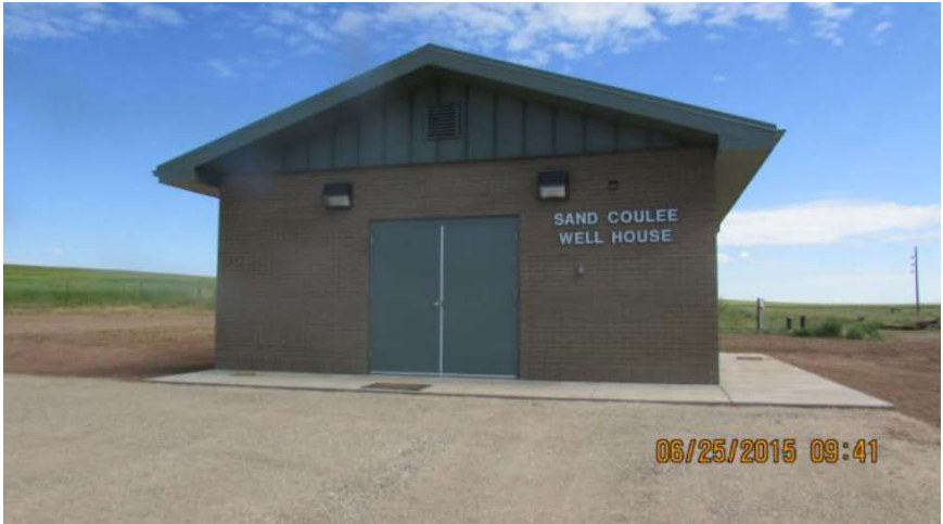
Completed well house in June 2015
