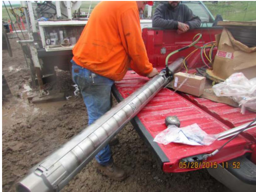
25 HP 160 GPM pump installed in Well #5 in May 2015
